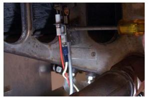
Removing electronic/standing pilot assembly.
